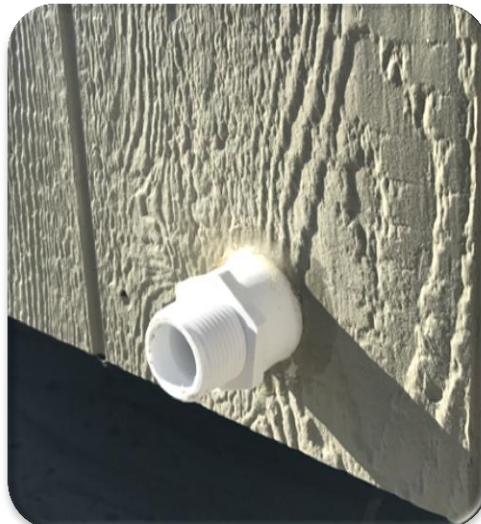
Water Heater Drain Line Installed
